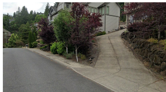
Example of curb-adjacent sidewalk. This arrangement would be allowed in areas of steep slopes or wetlands
