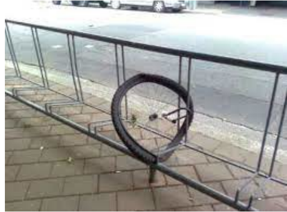
Bicycle racks of obsolete or inadequate designs may not protect the bicycle against damage or theft.
