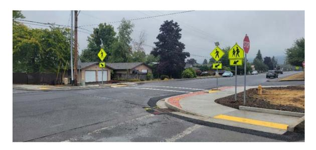
A project to improve the pedestrian crossing on La Creole Drive at Academy Street was recently completed. The project included the construction of new sidewalks with curb extensions (to reduce the width of the street pedestrians need to cross), new ADA ramps, solar-powered pedestrian-activated crosswalk flashers, and signage.
