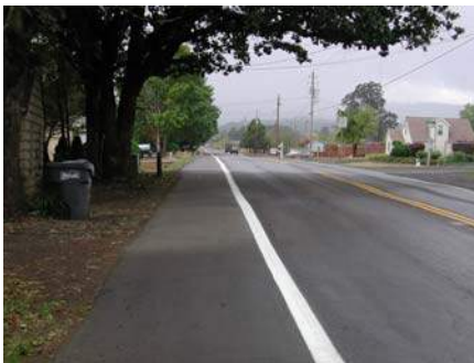
A 7' shoulder on the south side of W Ellendale Avenue west of SW Levens Street..
