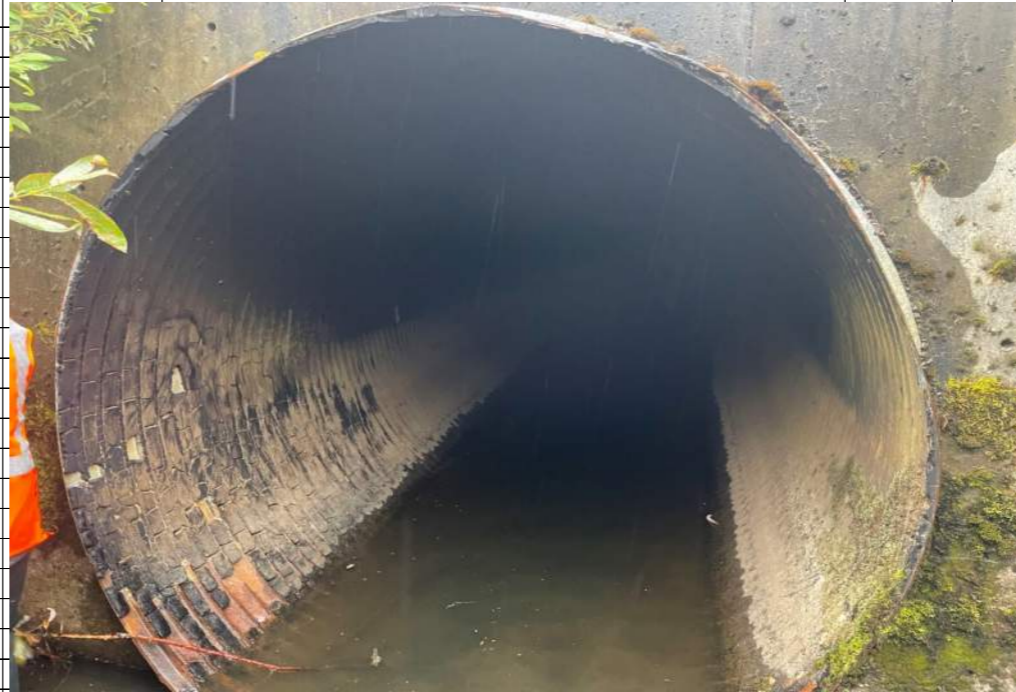
Left Upstream Culvert
